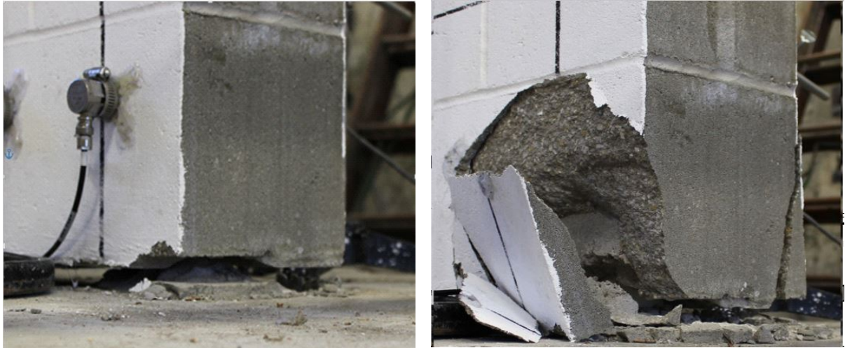
(a) Separation at the Bed Joint
